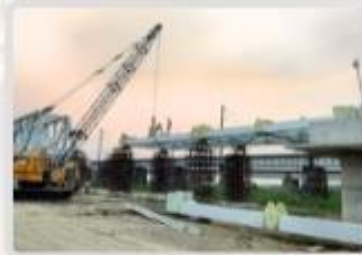
Bridge Construction & Fabrication
