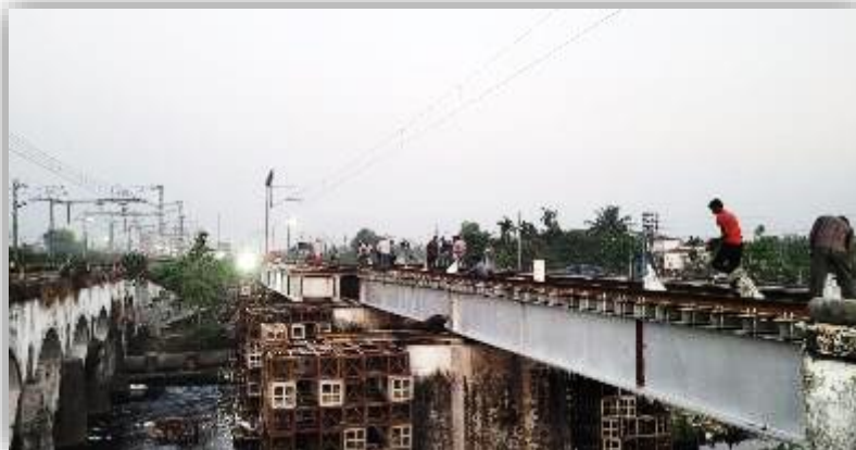
BRIDGES OF NFR2 (NEW JALPAIGURI)
